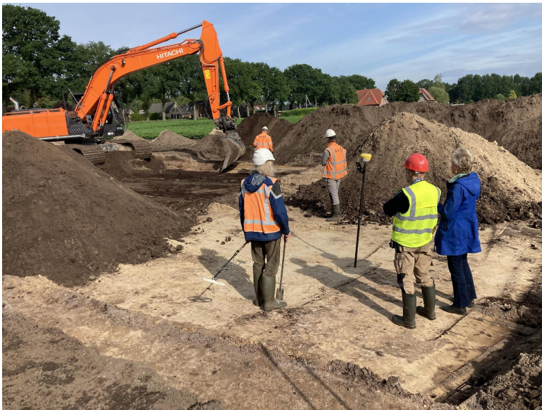
During the excavation
